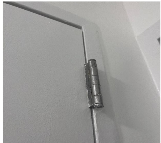
Eastchester Gardens: Stripped paint and rewelded hinges to existing frame and door
