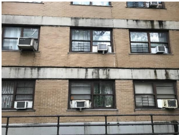
Existing conditions: facade staining
