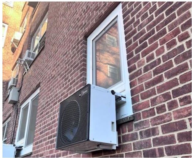
Clean Heat for All Program: Midea window unit with Intus window
